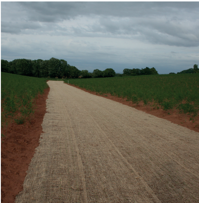
Figure 3. Bespoke GWW with jute geotextile to provide immediate protection from rainfall and runoff
